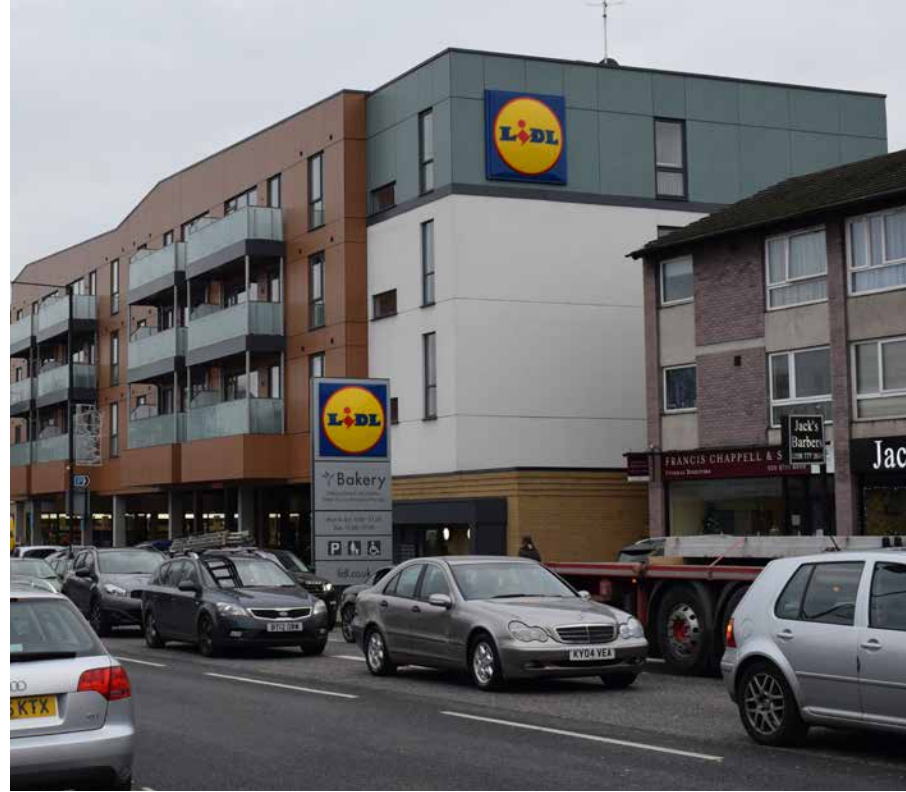
Figure 20 - Pedestrian access into car parking site
