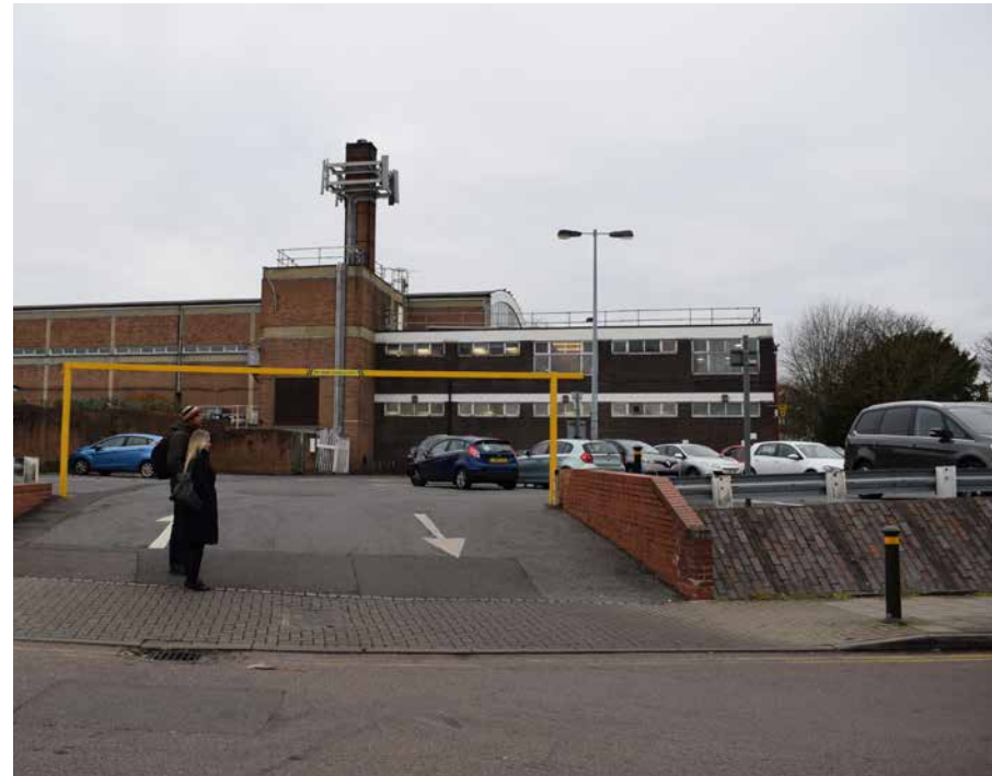
Figure 8 - View of the level change along Hawes Lane
