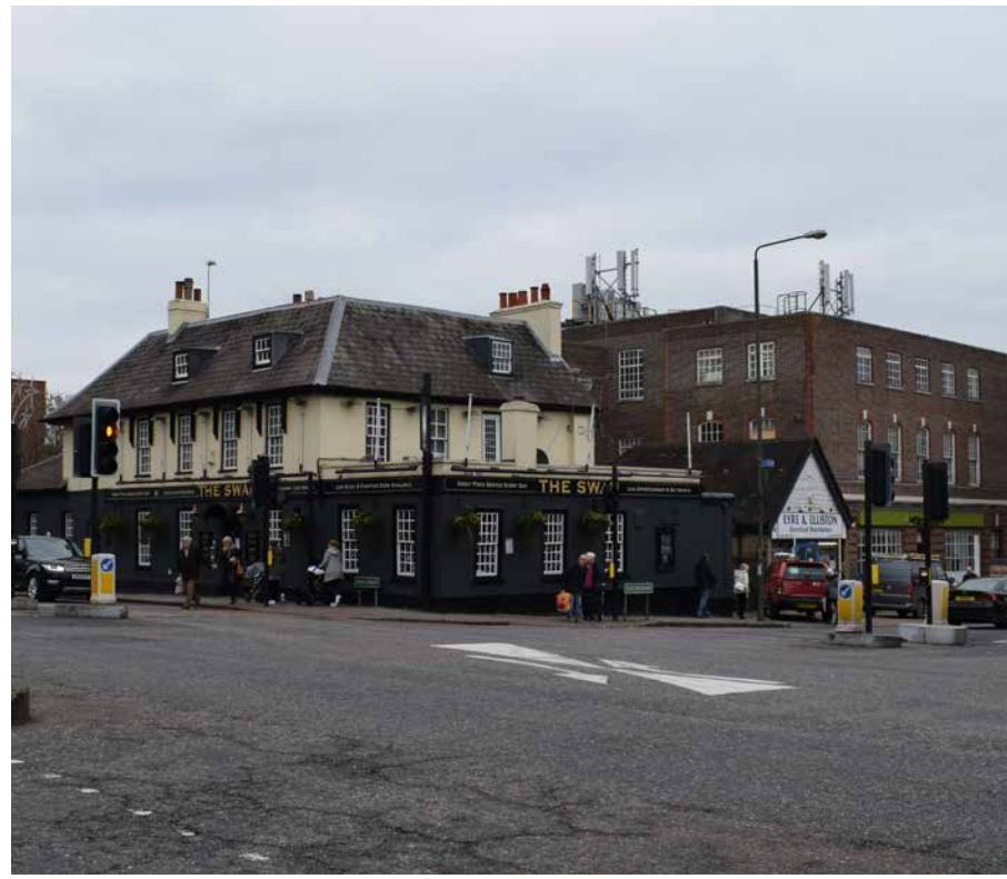
Figure 22 - Ground floor windows and shop entrances adjacent to WWL site
